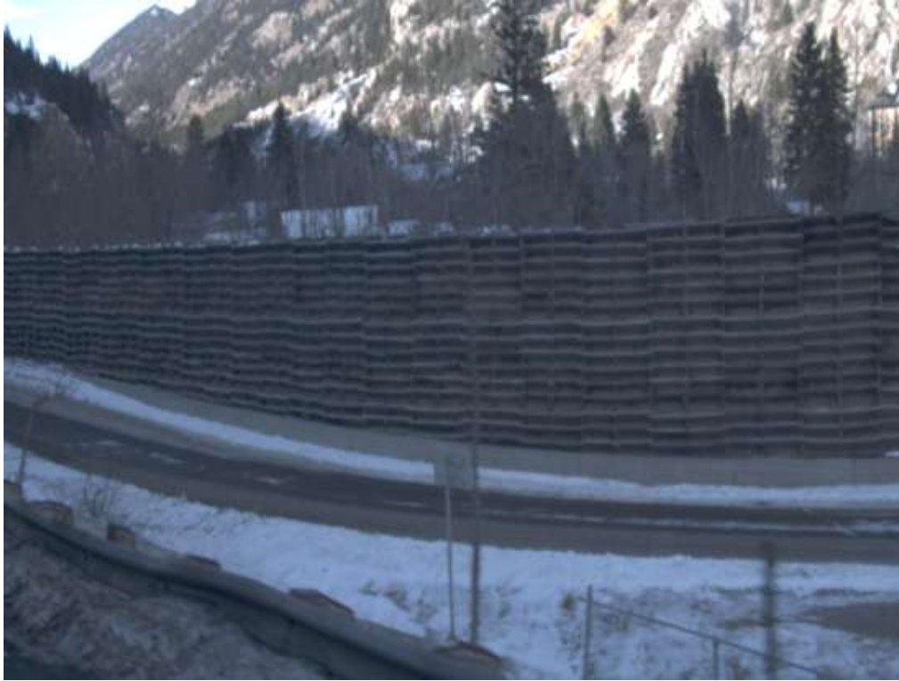
Fig. 15.1.13-7 Miscellaneous Sound Barrier Example
