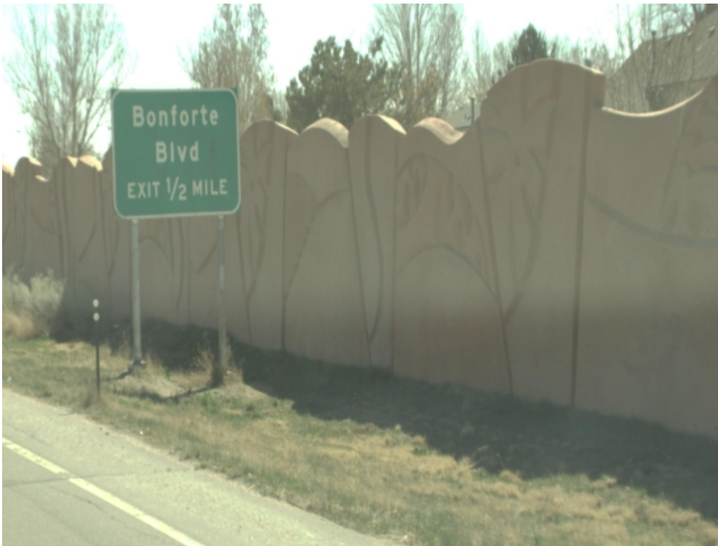
Fig. 15.1.13-8 Miscellaneous Sound Barrier Example 2
